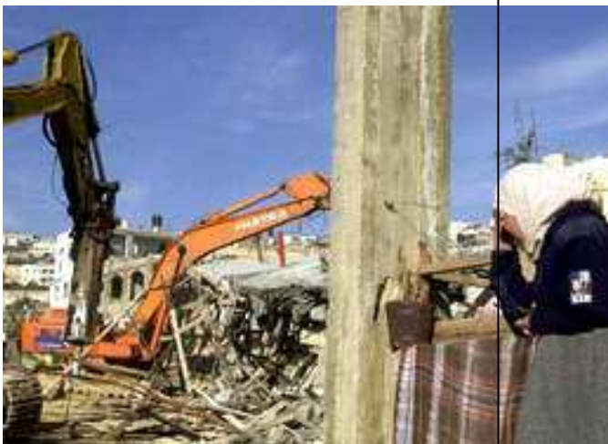
Figure 1. Original shot taken by Photographer of demolished Building.
